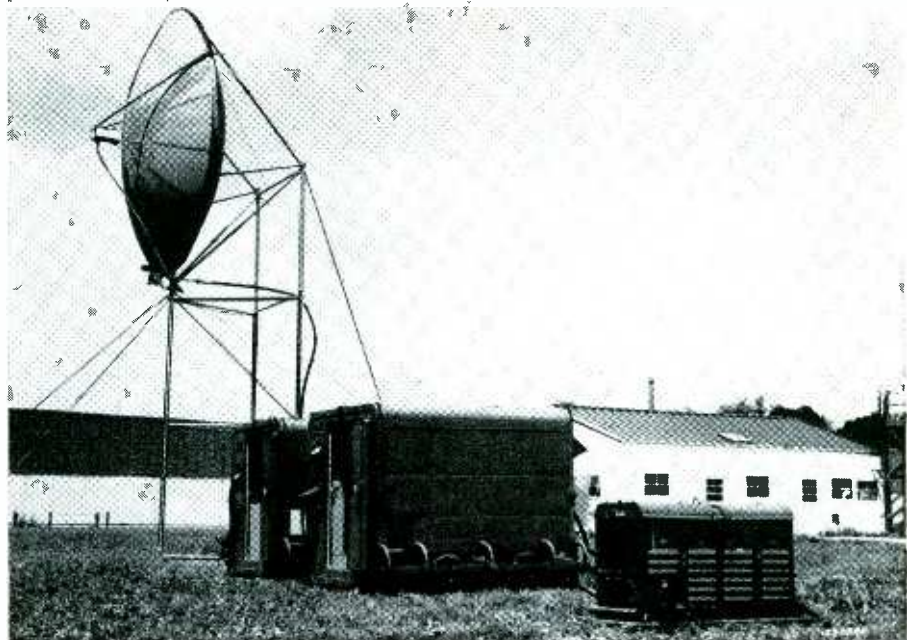
The terminal includes two air-inflatable antennas, a receiver-exciter shelter (left), and a transmitter shelter. All the equipment can be dismantled and packed for transportation in the two shelters except the portable generator (right of enclosures).
